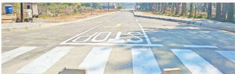
The recently completed upgrade of Lilanda Avenue, before and after, from gravel to asphalt has improved access for residents, businesses and investors.
